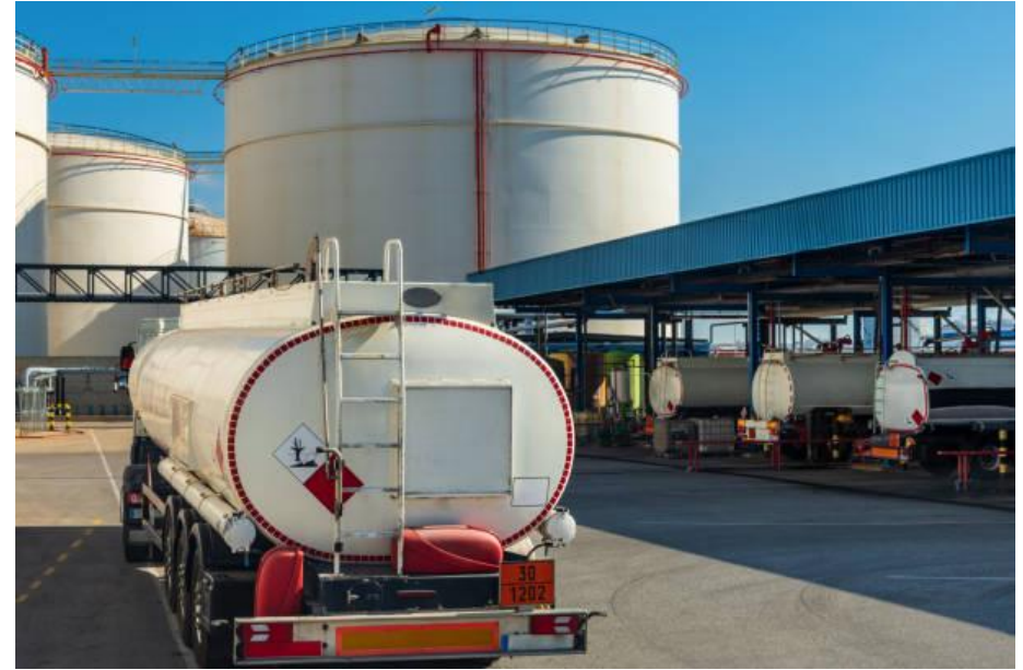
Fuel terminal truck rack with multiple fuel tanks
