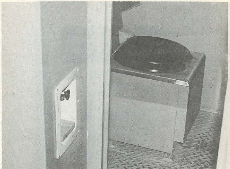
Fig. 3 — Typical Application of Incinerator Type Toilet
