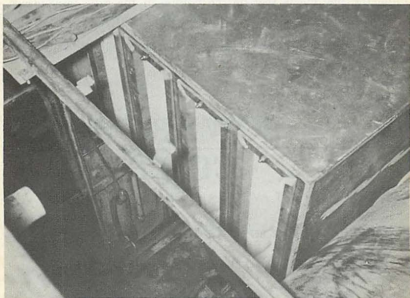
Fig. 7 — Completed Application of Housing and Filter Elements
