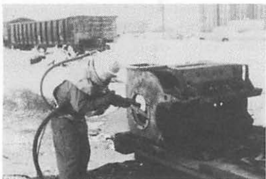
FIG. 23 — USING CORN COB GRIT BLASTING
