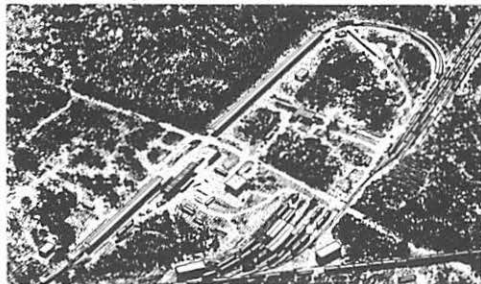
Aerial view of plant.
