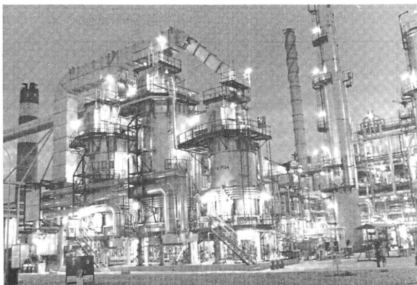
Figure 11 – Lubricants Refinery (courtesy Emerson Refining Company)
