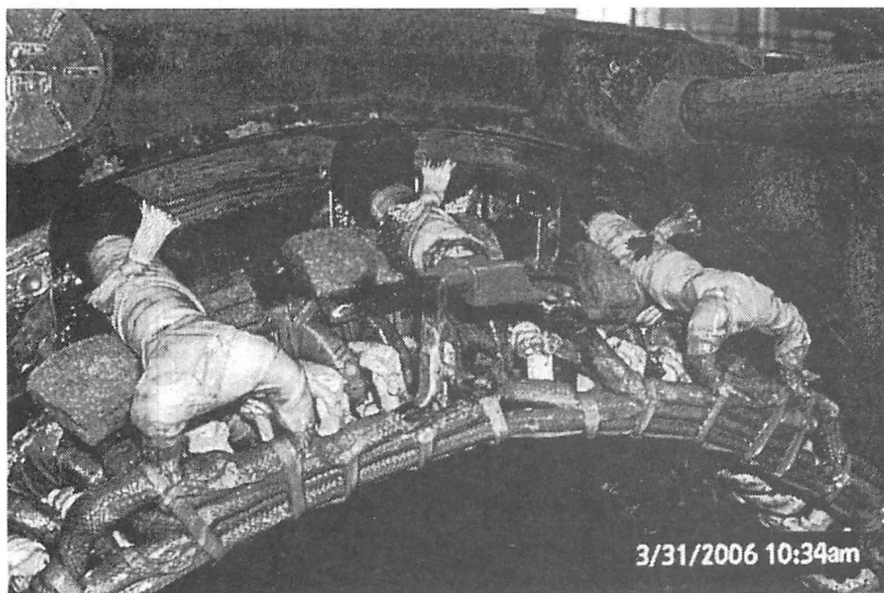
Figure 13 - Repaired Motor Cable Connections of Half Open Motor
