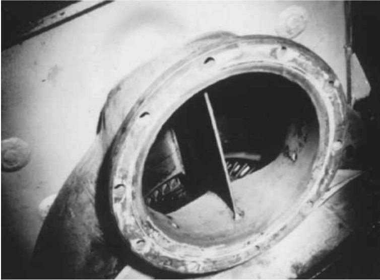
Figure 3: Turbine blade inspection through exhaust inlet scroll
