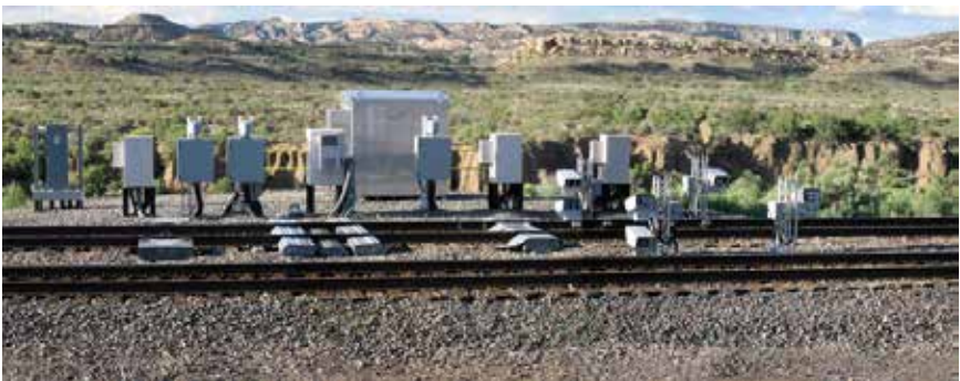
A typical multisystem detector site (All vision based system located at Gallup, NM on a BNSF track)
