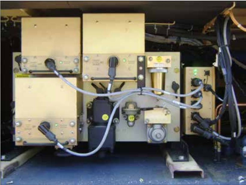
Figure 3. A 184 day maintenance interval brake system.
