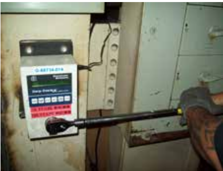
Figure 9: Proper Wrench Handling with Two Hands
