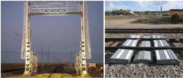
Figure: TrainView and CSCView systems installed at TTCI and BNSF
