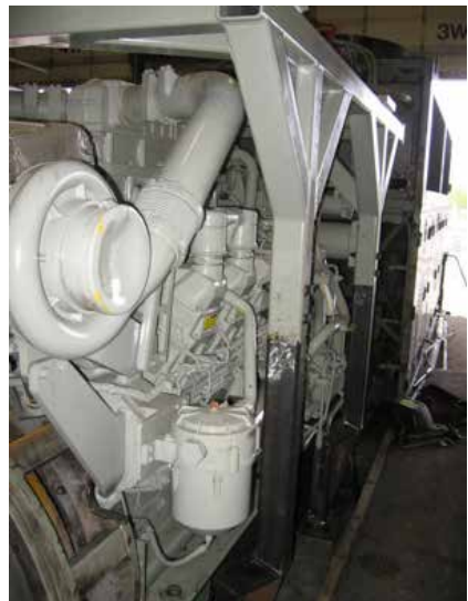
Figure 5: DPF Support Frame – Note; End Bracing for Structure Not in Place
