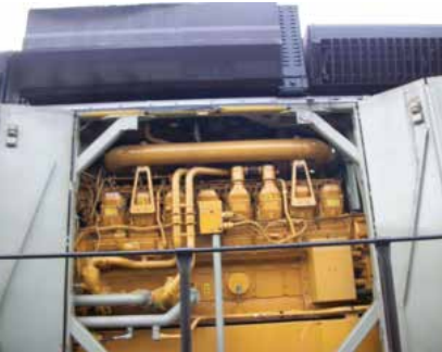
Figure 18: Engine with DOC/SCR above Engine
