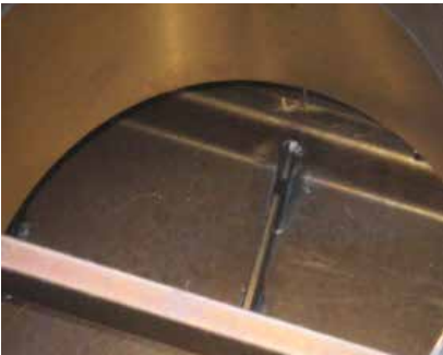
Figure 8: Inside of Exhaust Stack and DPF after Initial Testing July, 2011
