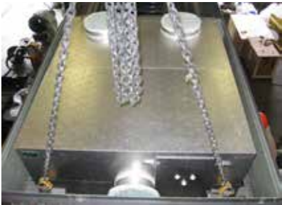
Figure 7: Installing DPF with Top Car Body Hatch Removed
