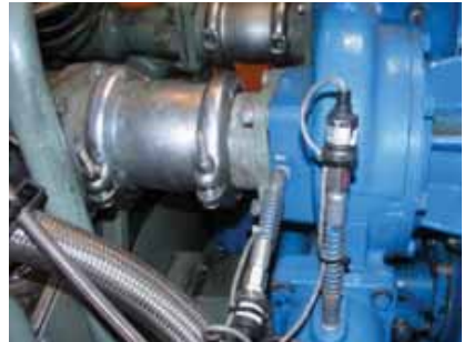
Figure 6 – Water pressure transducers, flex mount
