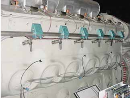
Spark ignited natural gas on an EMD engine
