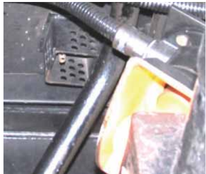
Figure 4 – Ambient temperature transducer, original location
