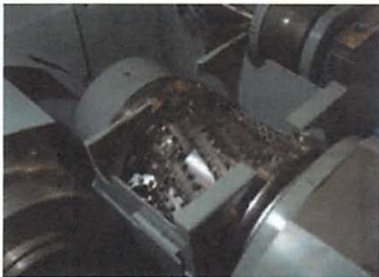
Installed Milling Cutter
