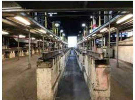
Figure 4. Raised Rail Pit
