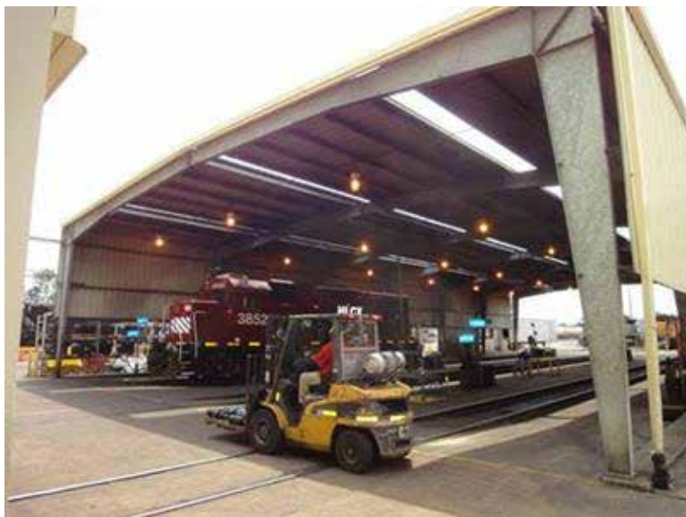
Figure 10. Outdoor Startup Shelter
