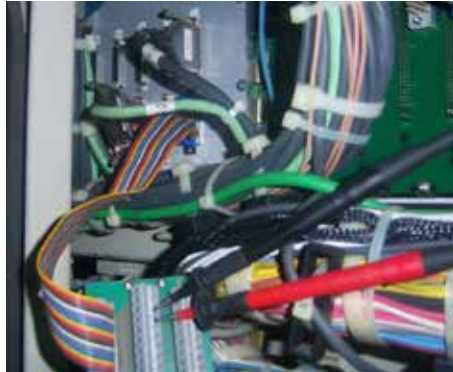
Figure 16. Checking the SD4 Cable
