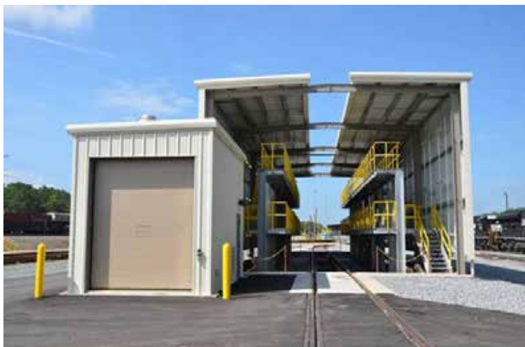
Figure 9. Three Tier Wash Station
