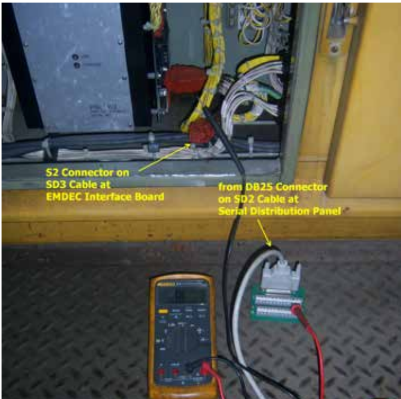
Figure 15. Checking SD3/SD2 Cable
