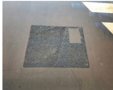
Missing Locomotive Label
