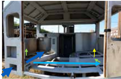
Figure #10. The large to small arrows illustrate the air flow from large to small. Each time the air is forced to turn, the pressure drops resulting in less air velocity.
