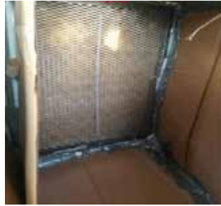
Figure #9 Updated filter inlet (971 CFM)
