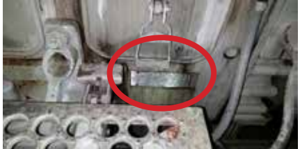
GE EVO Engine Location Under Crankcase Door – Left Rear Side
