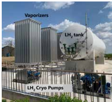
Figure 5: LH 2 Fueling System
