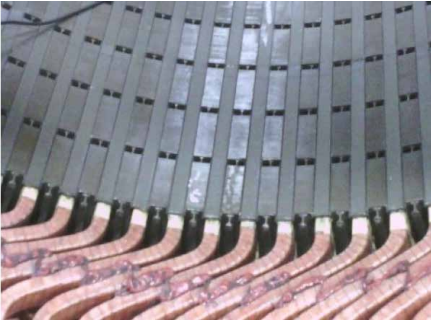
Figure 6: Core laminations being tested during core loss test.
